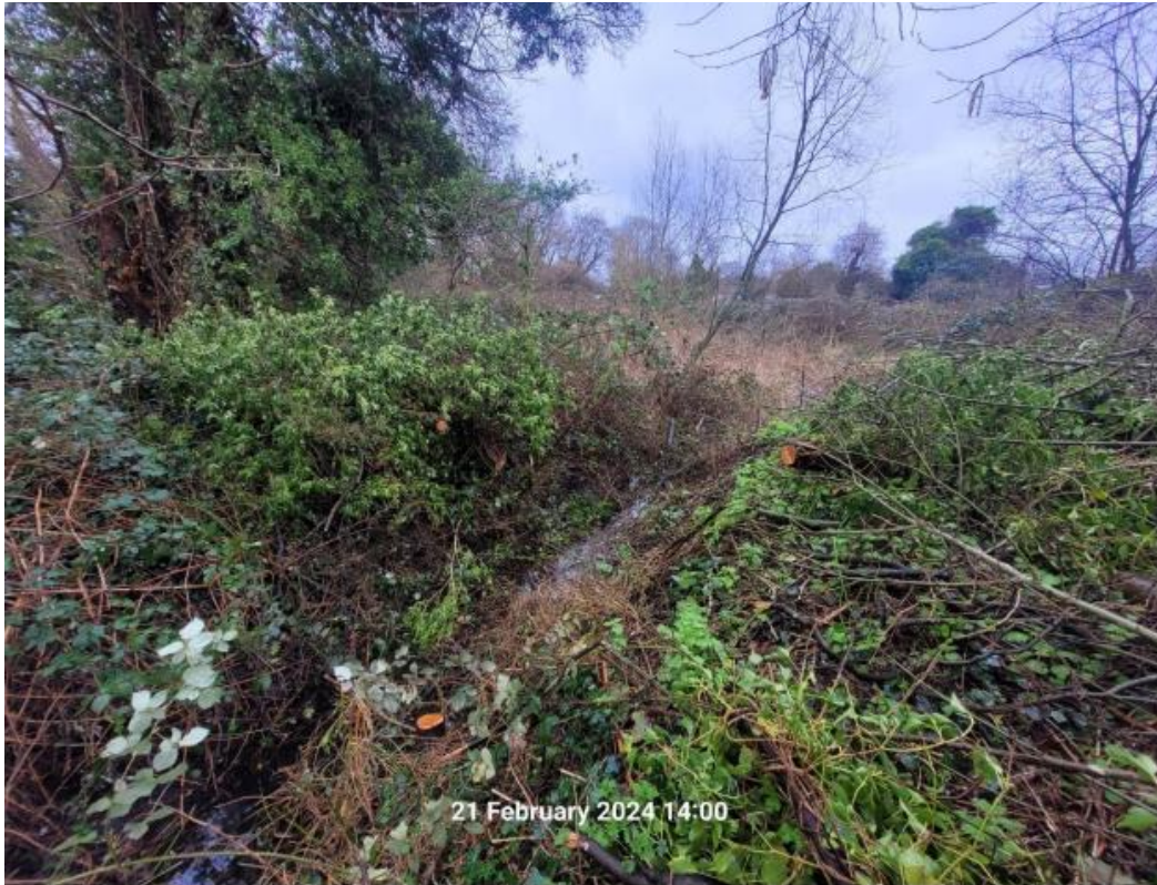
Inlet channel bottom – towards wetland
